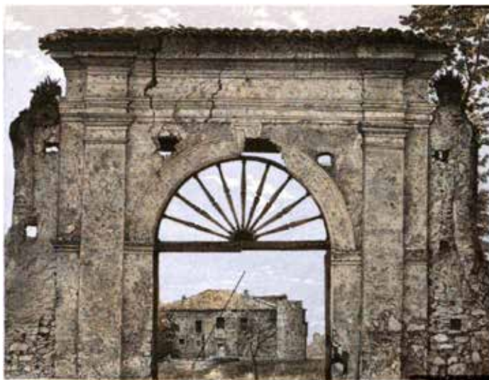
THE PORTE COCHERE, ON THE MILITARY ROAD, VILLA GARUSSO, NEAR AULETTA.
